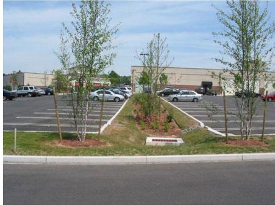
▼ Stormwater runoff flows into a green street facility.
